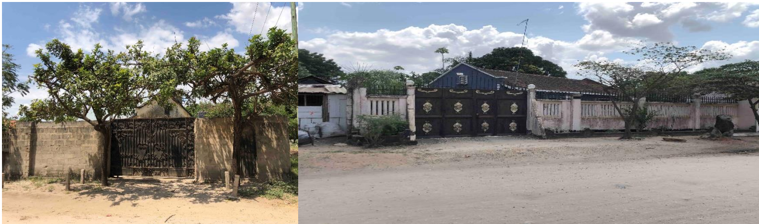
Figure 4: Existing residential buildings along Basri Road
