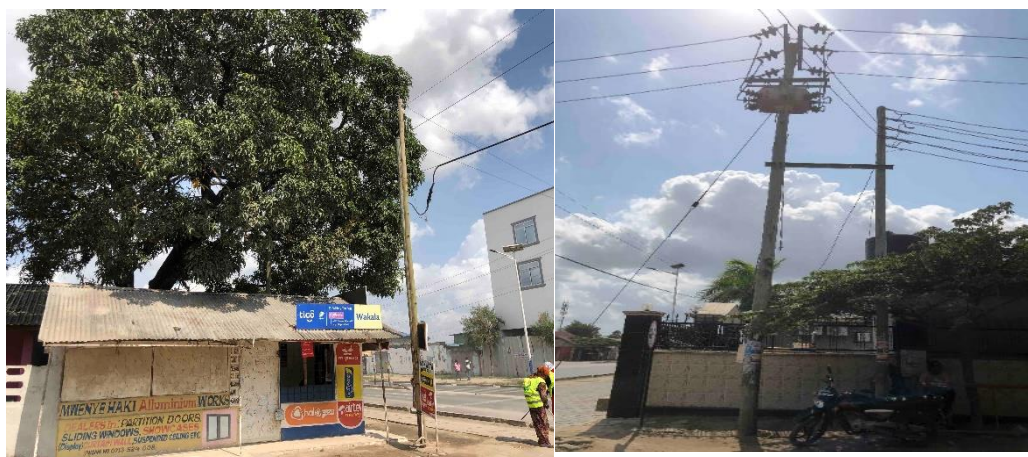
Electric pole adjacent to a residential house fence RHS
